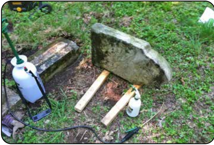
Figure 1. Necessary tools and the base and headstone ready for cleaning.
