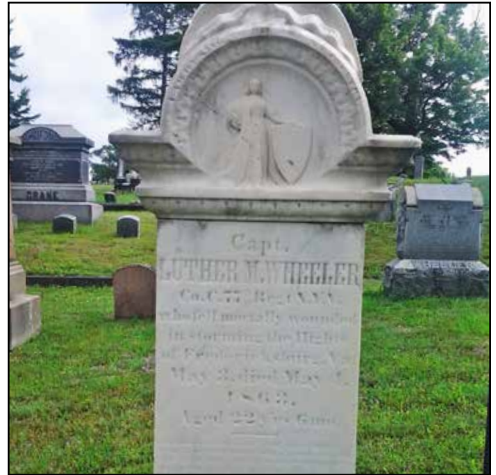
The correct use of D/2 for cleaning grave stones can be very dramatic. After use the stones details are very oveous on Capt. Luther M. Wheeler's stone.
