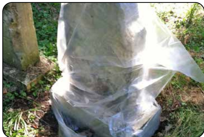
Figures 7. Grout curing step.
