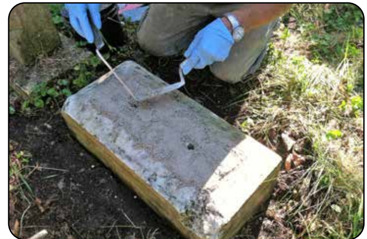
Figure 4. Placement of grout.
