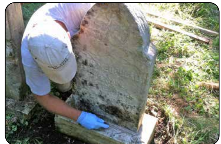
Figure 6. Finishing touches to the grout.
