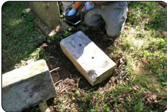
Figure 3. Clean, pins straightened, pinholes cleaned out and ready for grout.
