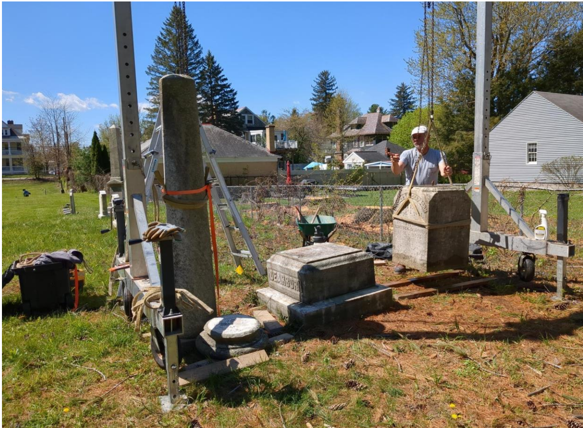
Figure 2. Disassembling the McIntosh Obelisk with a Gantry Crane
